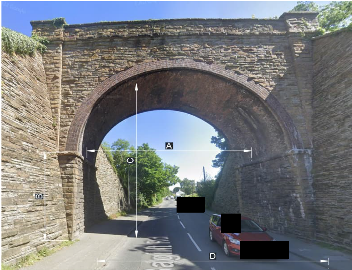
Figure 3.5 | Grade II overbridge
